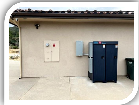
Battery and inverter enclosure supporting a 24 panel 9kW system
